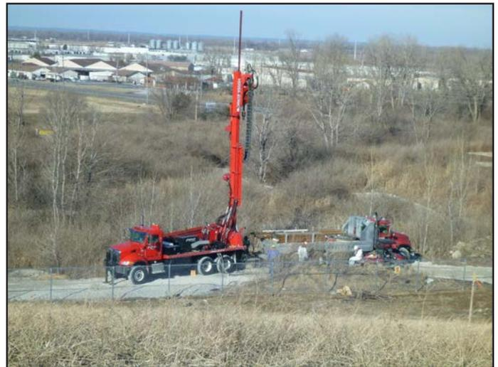
Drilling and core sampling to locate an isolation barrier between West Lake Landfill and Bridgeton Landfill is going on for the next several weeks. (U.S. EPA photo)
